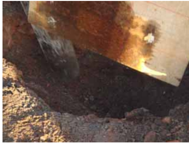
Shuttering for the postcrete
