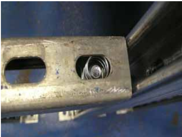
Fittings called Zebedee's were used to join pieces of unistrut together
