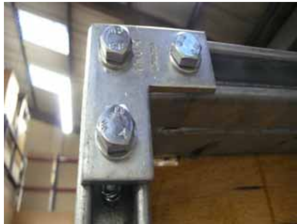
M12 bolts were used to secure the plastic to the unistrut
